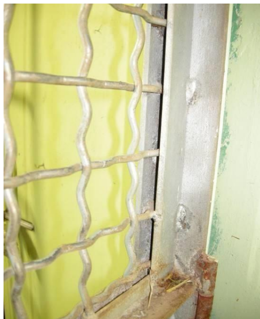
Fig. 8 Wave mesh welded between steel profiles.
