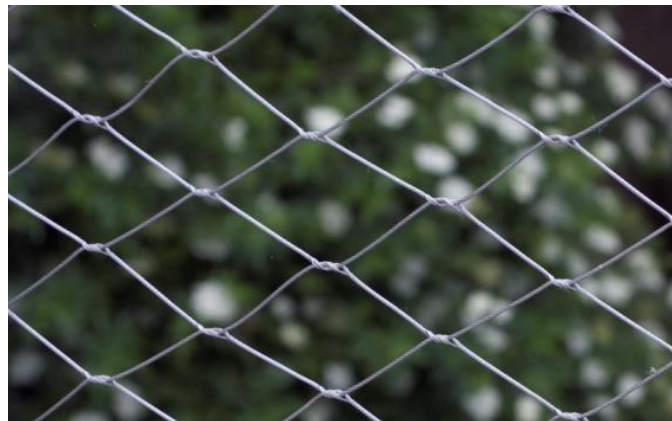
Fig. 9 Woven mesh with interwoven cables
