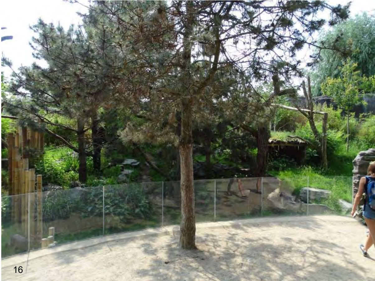
Figures 16-19: Different fencing options for tufted deer. Glass provides a nice viewing area for the visitors. Bamboo can be used for a decorative effect on closed walls. Closed walls and covered fencing are preferred over open fencing. Electric fencing should be only supplementary. Fig. 16: Zoo Leipzig Fig. 17: Parc Animalier d’Auvergne Fig. 18, 19 & 20: Zoo Heidelberg
