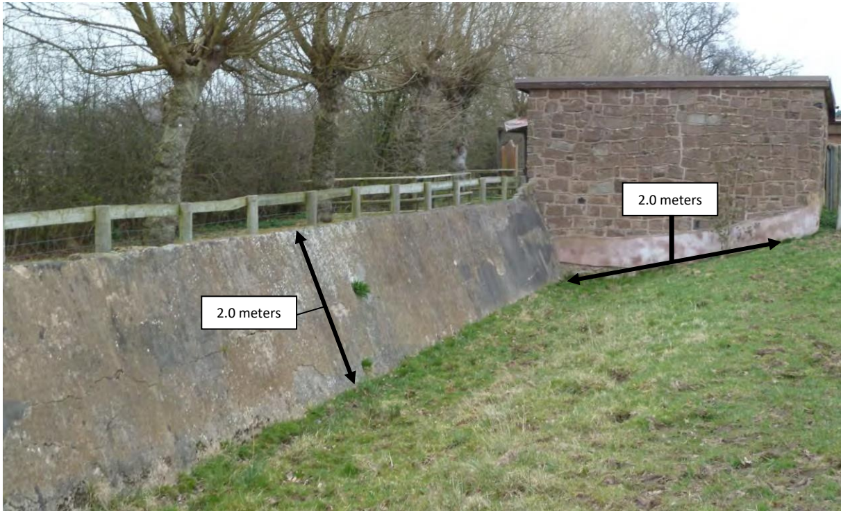
Figure 2.3: A 2.0 meter high concrete barrier on a gently sloping ditch.
