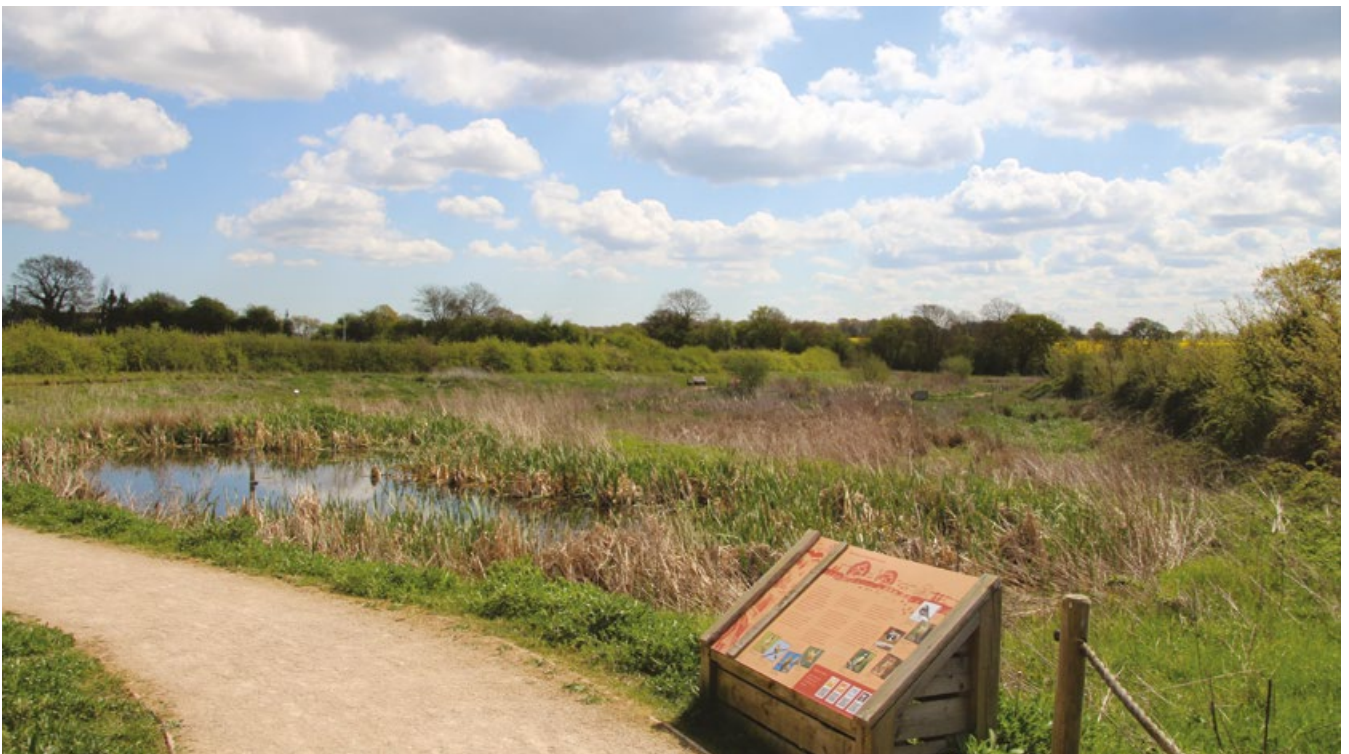
Water management is a focus for operational sustainability in EAZA zoos – one example is this reed bed filtration provided by Twycross zoo's constructed wetlands, which also provide a habitat for local species © Nicola Williscroft
