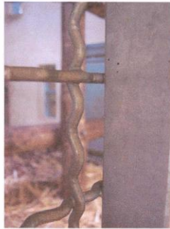
Mesh welding to frame (intermediary)
