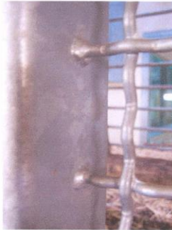
Mesh welding to frame (terminal)
