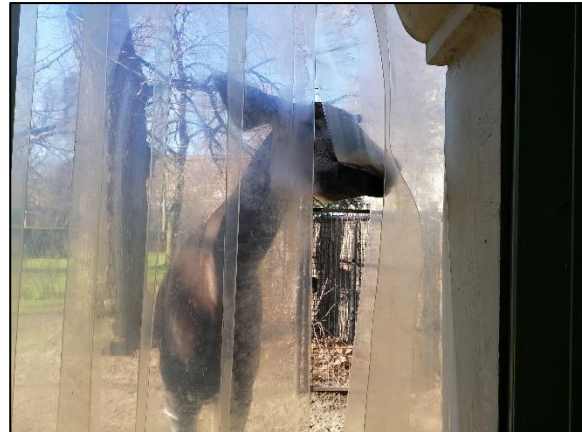
Figure 48 – Plastic strips on the doors are a good option to keep the indoor facilities insulated from cold weather while still allowing the animals to enter and exit the facility. ©Antwerp Zoo / Location: Antwerp Zoo
