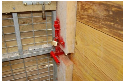
Figure 26: Security system to allow keepers to go in the outdoor enclosure with padlock and unique key © CERZA zoo
