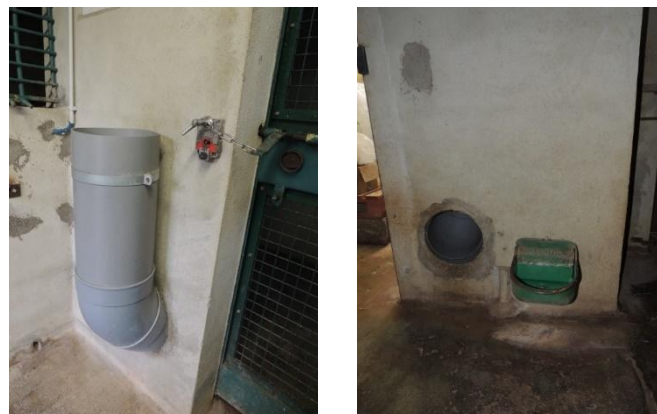
Figure 36: Food distribution gutter system on the keeper side (on the left) and in the enclosure (on the right) at Obterre zoo © P. Roux
