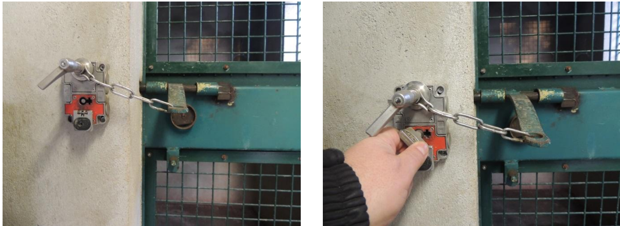
Figure 30: Latch of the door locked (on the left) and turn the "unique key" to release the latch (on the right) © P. Roux, Obterre zoo
