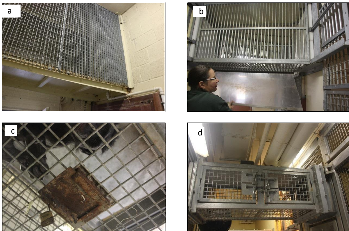
Figure 28: Designs for overhead tunnels in bonobos. a: Solid bottom tunnel with water drainage (Planckendael – Jeroen Stevens); b: Wire bottom tunnel with plastic sheet protection (Apenheul – Jeroen Stevens); c: Small door in tunnel bottom for ultrasound inspections (Milwaukee Zoo – Jeroen Stevens); d) Side doors to be able to remove sedated bonobos from the tunnel (Milwaukee Zoo – Jeroen Stevens).
