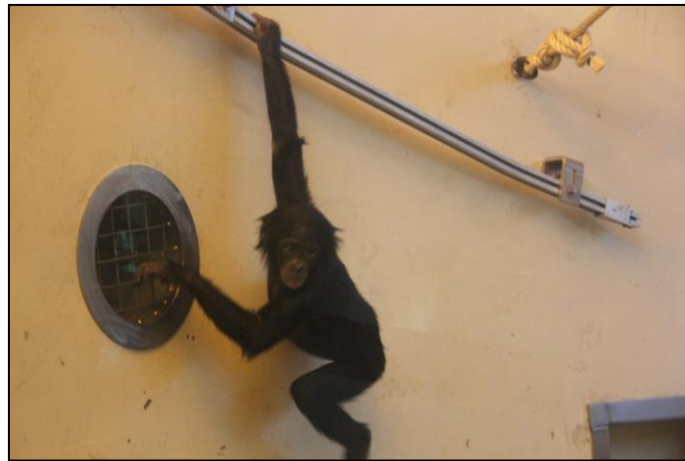
Figure 37: Air vent installed to allow air circulation between adjacent enclosures also when the full slides between the enclosures are closed off (Apenheul – Jeroen Stevens).
