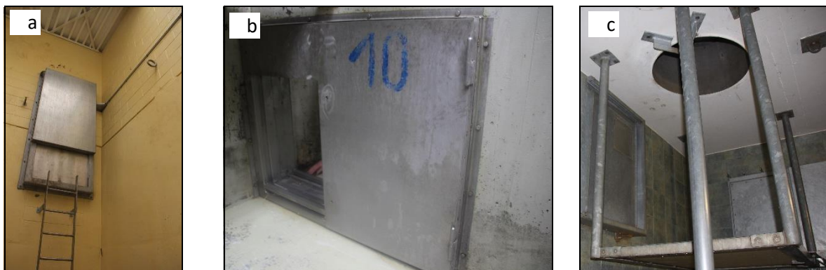
Figure 24: Different sliding doors in bonobo exhibits. a: door that slides in a vertical plain (guillotine door) (Milwaukee Zoo - Jeroen Stevens); b: door sliding in a horizontal plane (Cologne Zoo - Jeroen Stevens); c: sliding door in the ceiling connecting enclosures that are on top of each other (Leipzig Zoo – Jeroen Stevens).
