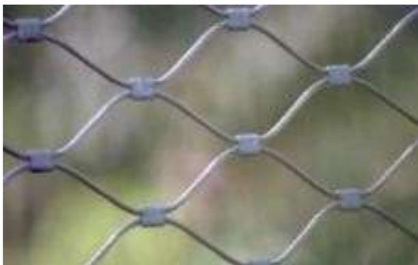
*Figure: 15: Ferrule type cable mesh.*
