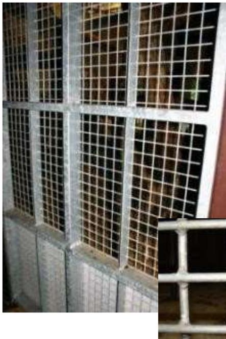
Figure 11: Welded mesh
