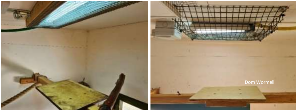
Fluorescent UVB tubes positioned on the ceiling of the inside area of an enclosure.
