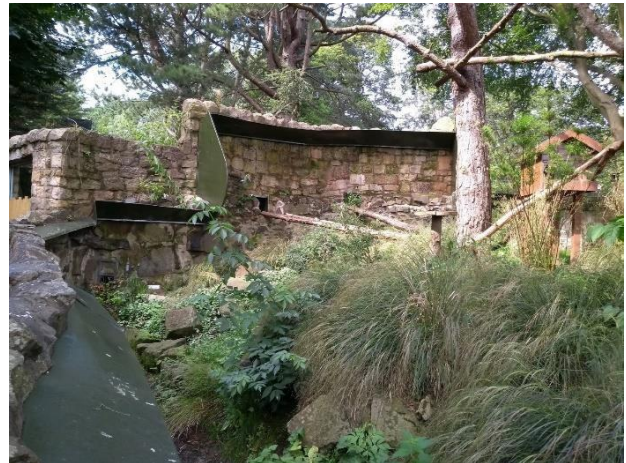
Picture 7: Wall with overhang Zoo Zurich (photo by Wietse Verwer)
