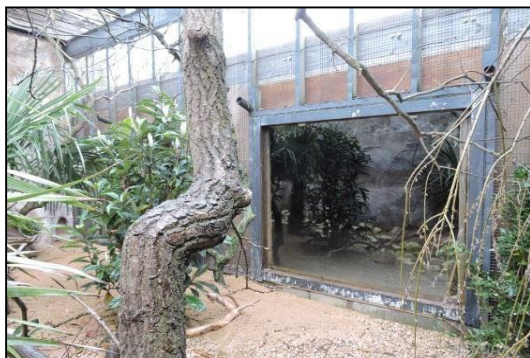
Wood lined with sheet metal / wire mesh
