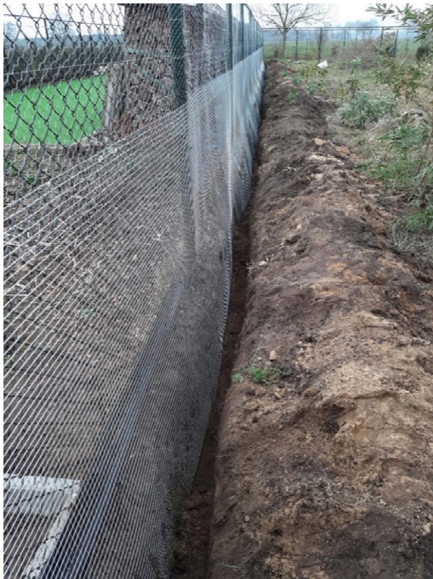
Fig. 18: Metal mesh dug into the ground © Jan Dams
